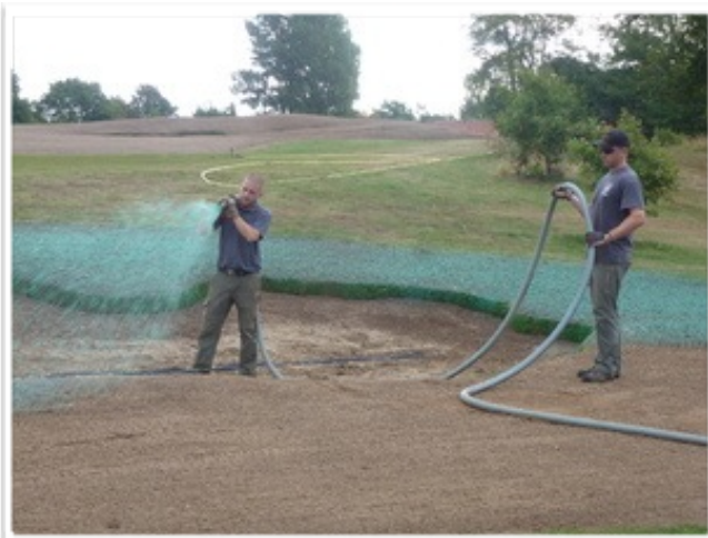
Applying the hydraulic slurry of seed
