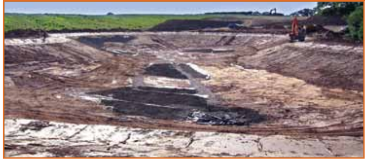
Lake & Reservoir Construction & Lining
