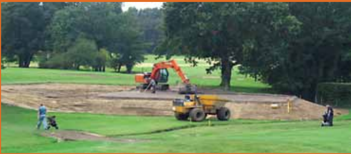
Tee Reconstruction & Laser Grading
