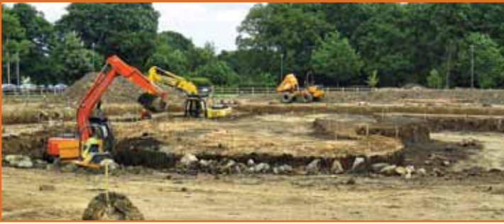
New Build Golf Course Construction
